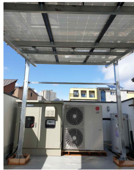
<전전화주택(all-electric system) 에너지공급시스템(PV+ESS+Heat-pump)>
